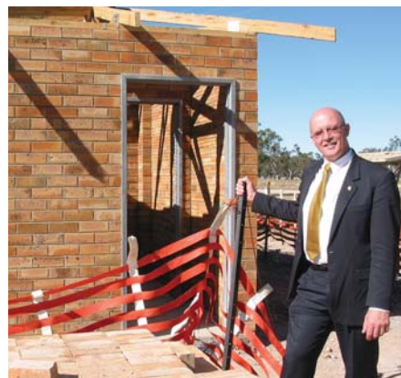
Peter Draper MP at the Redbank rest area on the Oxley Highway during construction.
